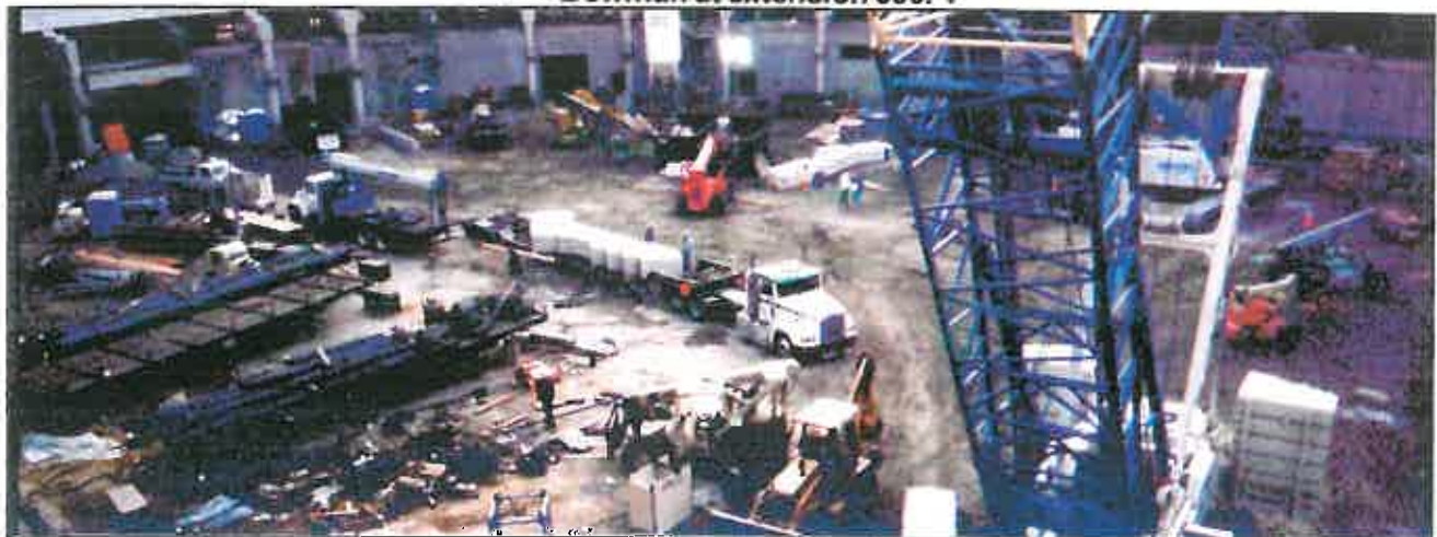
DTI truck "center court" inside the future arena.
