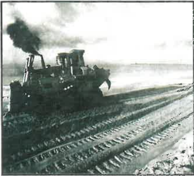
DTI's dozer digs in against the tide.
