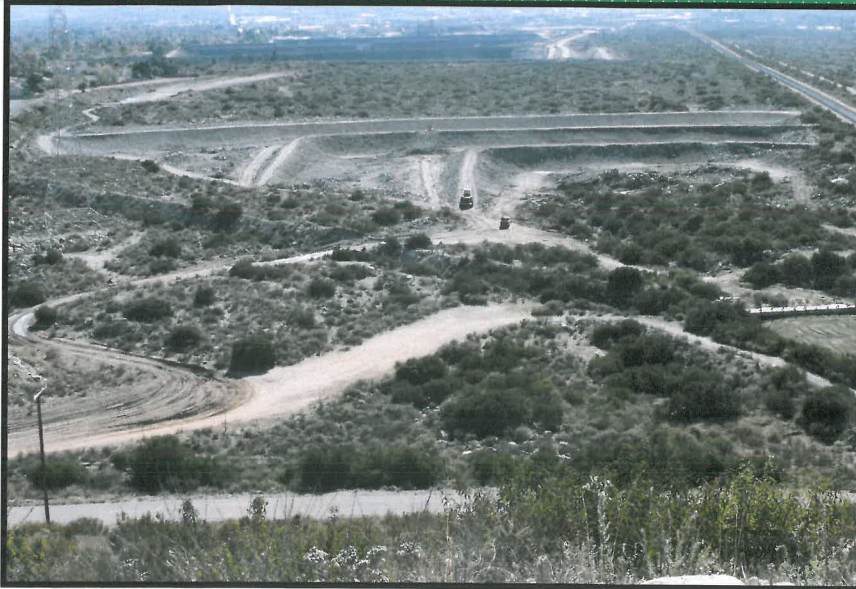
Pictured above is the Dalton Team at work expanding the berms that is being used to retain rain water and run off from the near by hills.
