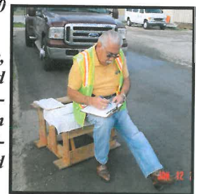
(Right) Our site Manager, Flash Imamura, keeps detailed notes of trucks used and tonnage delivered. His being on site allows our customer to adjust volumes of rock vs. sand during the day.
