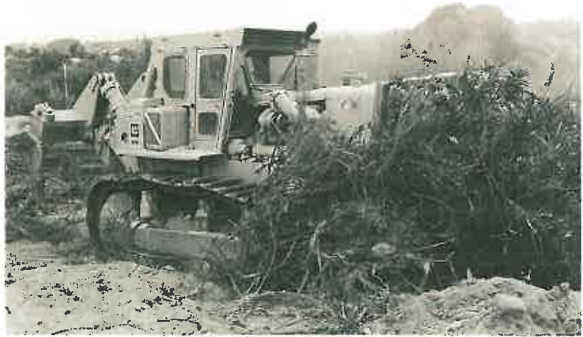
Grubbing is usually the first step.
