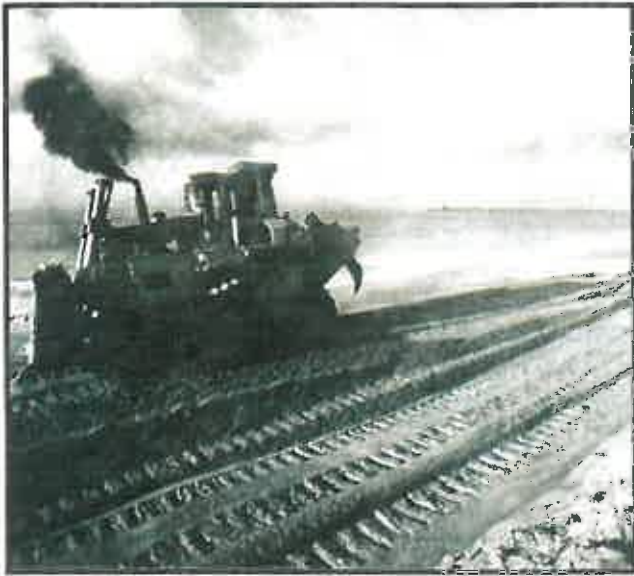
DTI's dozer digs in against the tide.
