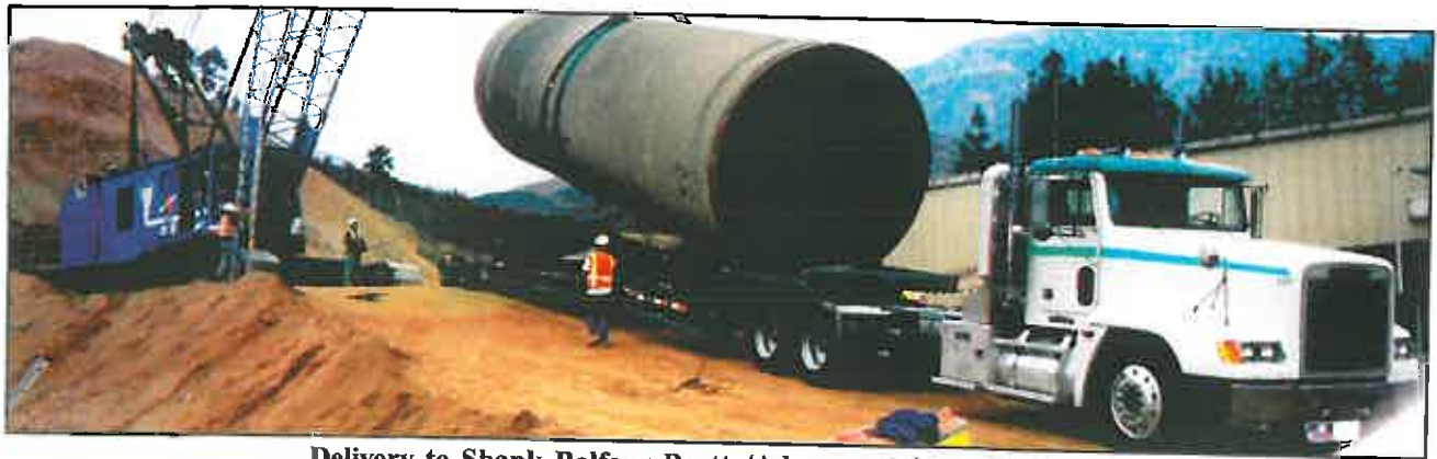
Delivery to Shank Balfour Beatty/Advanco at Arrowhead West
