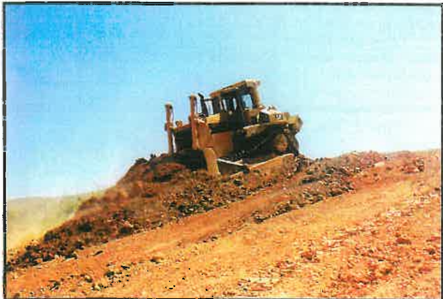
DTI's D8 efficiently pushing downhill.
